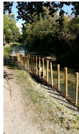
posts and hazel whips make a secure natural barrier to hold the widened towpath
