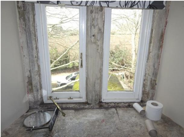
**Photo 3. Stone mullioned window with ovolo mouldings found on the attic floor**
